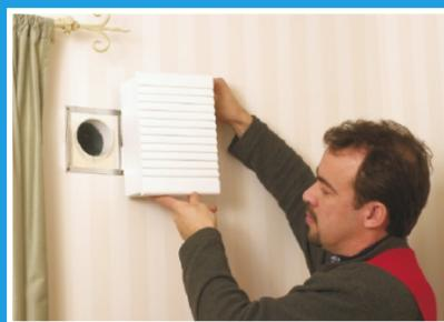
Install the unit on to the mounting bracket. The sealing at the back of the unit seals the unit against the wall surface. The unit has a power supply cord with a plug as a default for easy installation.
