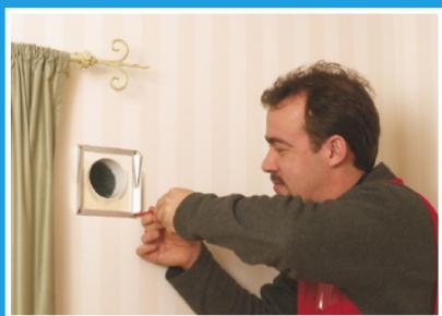
After installing the air duct and the outdoor louvre, the mounting bracket can be installed. In case the existing ventilation channel is wider than the unit, the mounting plate can be used.
