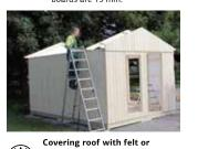
Roofing felt is the easiest and fastest way to protect the roof
