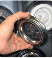
If the jets still fail to work, switch off the pumps from pump connections to avoid pressing out the water, carefully loosen the upper pump connection in order to discharge any air remaining in the equipment. Then tighten again pump connection and switch on the pumps. Switch pumps on and off several times, until jets start to work properly.
