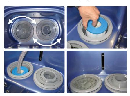
After draining, always fill the minipool through the filter canister. Otherwise air may remain in the pump and hinder it from creating a water circulation. Water level should cover filters at least by 10 cm.
