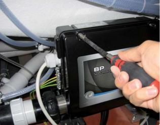
Remove the protective cover of the board, lifting the clampings with a screw-driver, as shown on the photos. The cover has 2 clampings in total.
