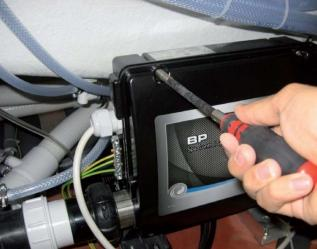
Remove the protective cover of the control unit. Unscrew the two screws located in the upper corner of the device by means of a screwdriver. Pull the upper edge of the protective cover away and lift the cover from the two fasteners at the bottom of the control unit.
